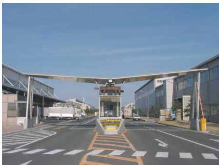
Tohoku Plant guardhouse building solar electricity generation system
