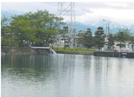
Kurobe facility cooling water collection pond
