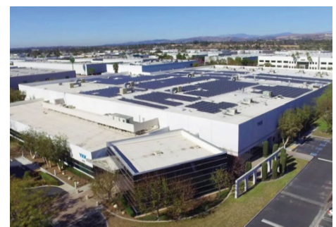
Example of solar power installation Anaheim Plant, YKK (U.S.A.) Inc.
