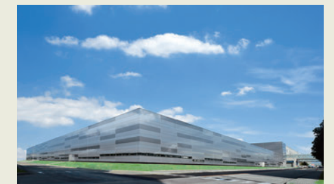
The Slide Fastener Machine Parts Plant
